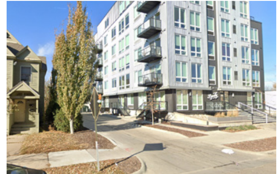
Example rear alley condition
