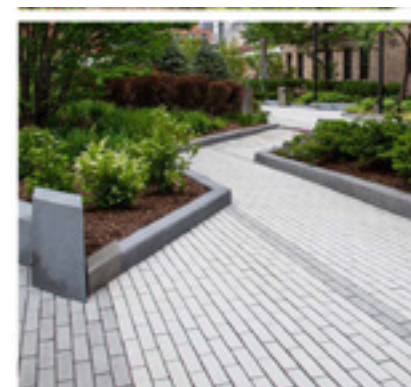
Permeable pavers and planting areas with underground detention
