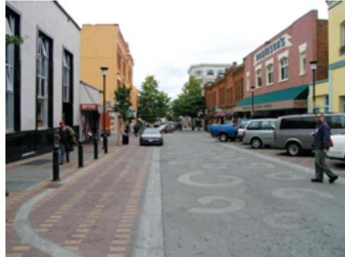
Example shared street in Victoria, BC incorporating angled parking and decorative paving
