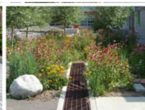
Permeable pavers and planting areas with underground detention
