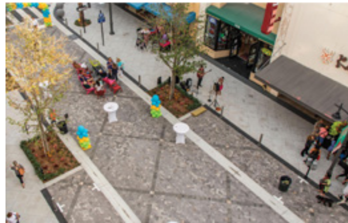
Example shared street (Clematis Street) in West Palm Beach, FL utilizing bollards and decorative paving to delineate space.
