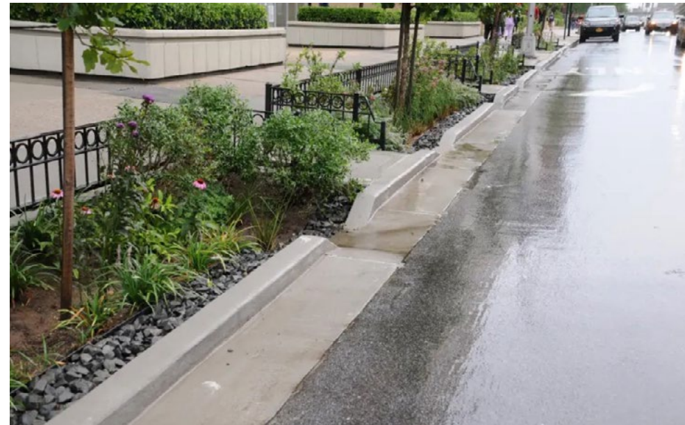
Street / Sidewalk Infiltration
