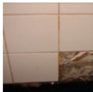
Mold growth under ceramic tiles in a bathroom. (photo, John Martyny, Ph.D.)
