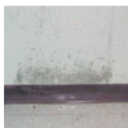
Mold on painted concrete in a school building. Rainwater is wicking directly through the concrete walls, and there is also condensation on the earth-chilled concrete (The floor is about 3 feet below ground level.) (photo, Terry Brennan)
