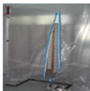
Full containment. (photo, Terry Brennan)
