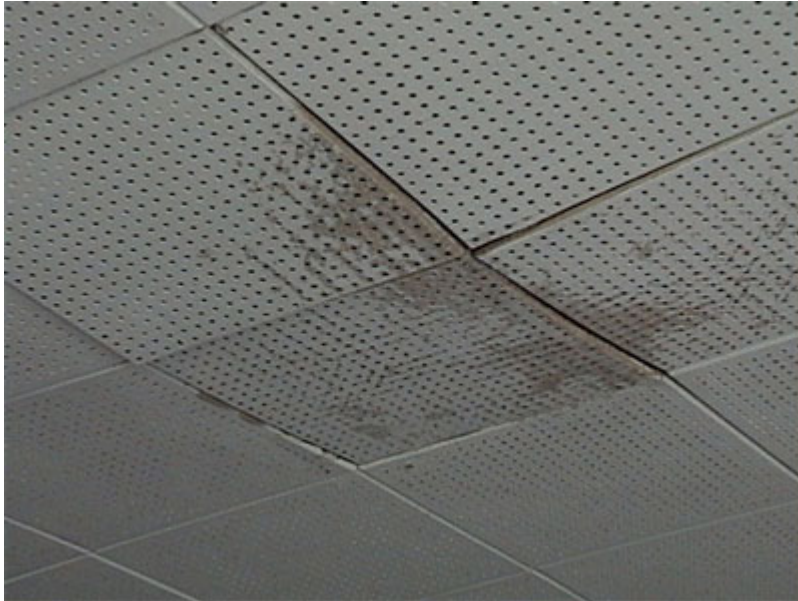
Water stains in basement. (photo, Terry Brennan)
