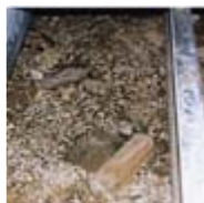
Mineral deposits on the surface of a dirt crawl space caused by chronic water problems. (This is not mold.) (photo, John Martyny, Ph.D.)
