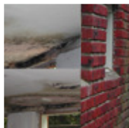
Mold on first floor beneath a through-the-wall air conditioner on the second floor. (photo, Terry Brennan)
