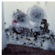
Moldy bedroom closet. Water condensed from the air onto the gypsum board. The wall is cool enough for condensation because there is a hole in the insulation and it is cold outdoors. (photo, Terry Brennan)
